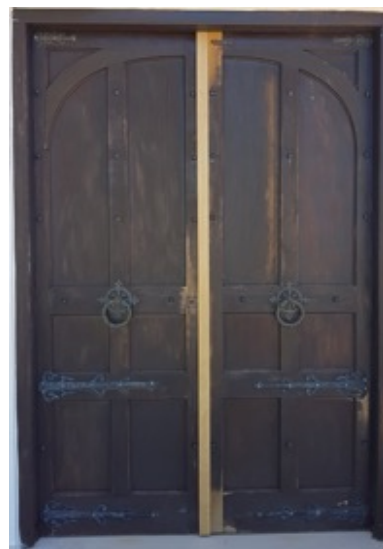
Door repair ready for painting
